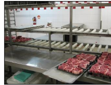
Upright fridge cabinets (and bakers' ovens) with continuous level floor surface allows stock to remain on trolleys and reduces resistance when pushing/ pulling
