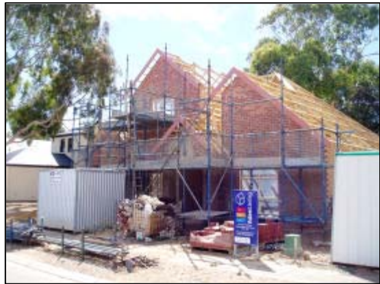
Compliant perimeter scaffolds on housing sites in Melbourne (above left) and Adelaide (above right). Below left: An edge protection system on a housing site in Sydney. Below right: Stair void protection on a housing site in Melbourne.
