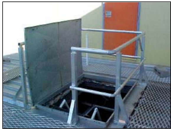
Above left: Roof edge full-perimeter guardrailing on an Adelaide housing site. Above right: Guardrailing on a commercial site in Melbourne for roof access by services installation trades.
