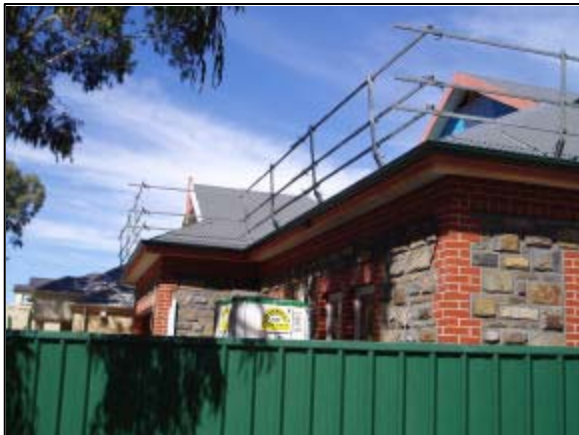
Above left: Roof edge full-perimeter guardrailing on an Adelaide housing site. Above right: Guardrailing on a commercial site in Melbourne for roof access by services installation trades.
