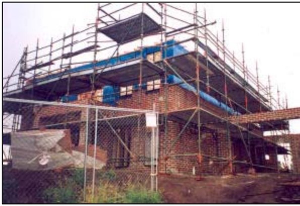
Compliant perimeter scaffolds on housing sites in Melbourne (above left) and Adelaide (above right). Below left: An edge protection system on a housing site in Sydney. Below right: Stair void protection on a housing site in Melbourne.
