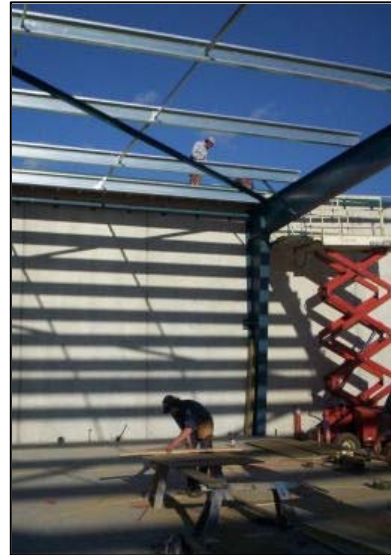
Small commercial sites were also targeted. Examples of lack of falls prevention at Townsville, Queensland, during roof plumbing work (above) and at a tilt-up factory project in New Zealand (right).
