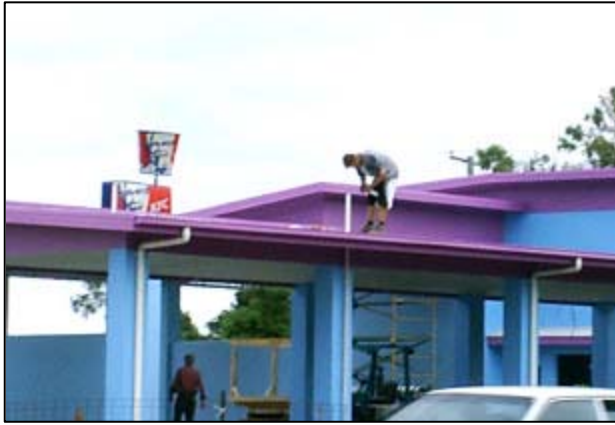
Small commercial sites were also targeted. Examples of lack of falls prevention at Townsville, Queensland, during roof plumbing work (above) and at a tilt-up factory project in New Zealand (right).
