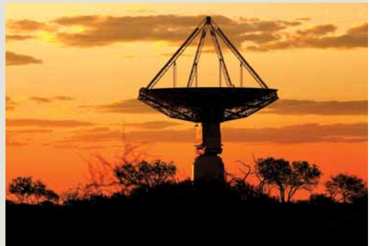
Innovation to develop renewable energy sources for radio astronomy is taking place in the State's Mid West.
