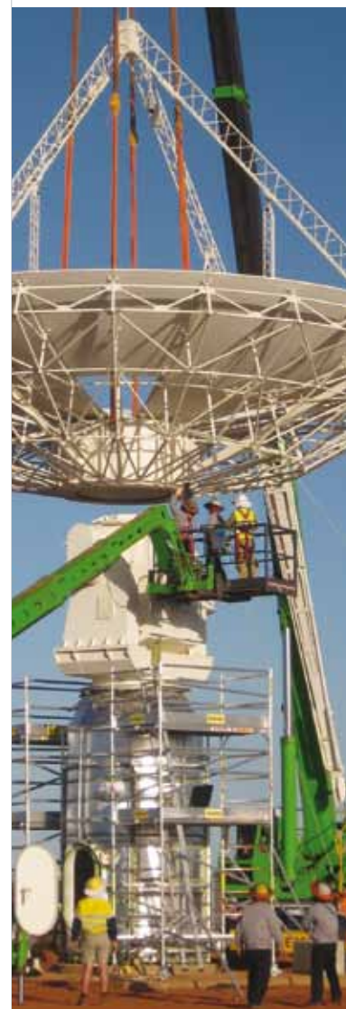
First ASKAP antenna under construction.
