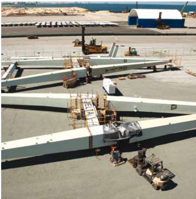
Fabrication of shiploader structure is well underway.
